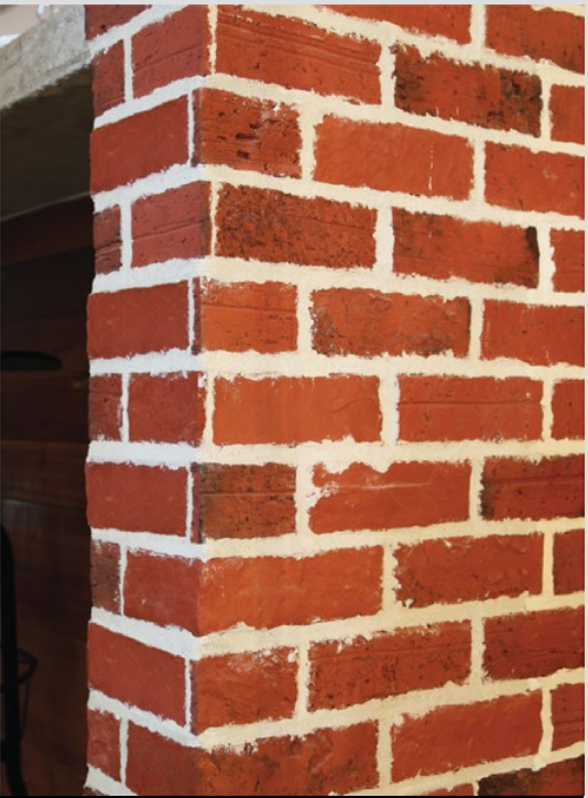
Application without Corner Brick
